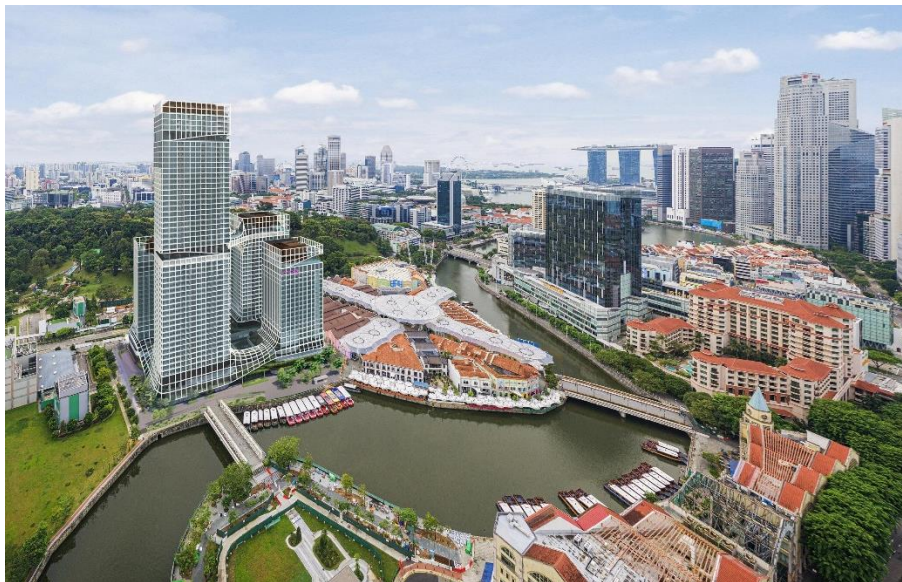
A day view of CanningHill Piers from the Singapore River (artist's impression)
